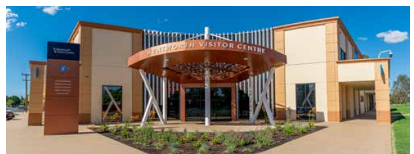
Wentworth Visitor Centre (Main Administration Office) 61 Dudley Street, Wentworth NSW 2610
